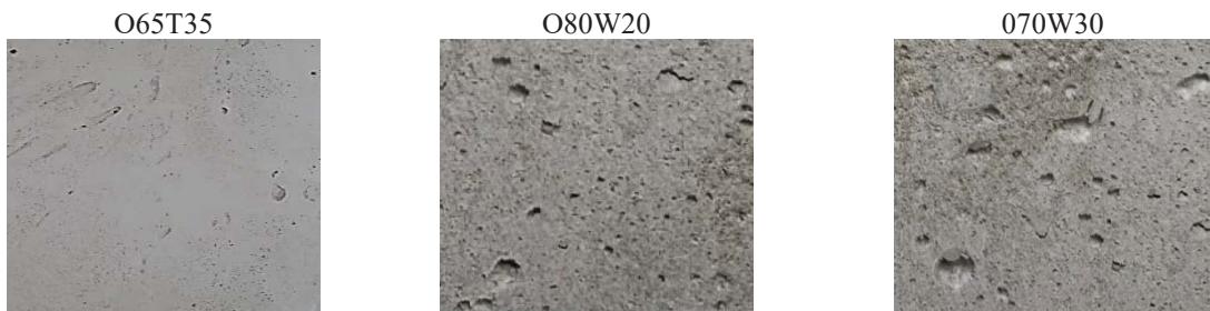
FIGURE 4. The surface condition of concrete specimens after demolding.
